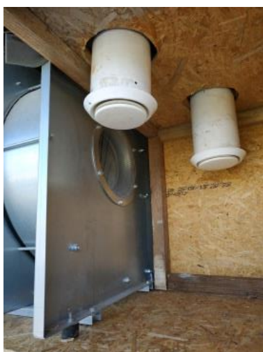
3.13. att. Ozona ģeneratoru kopskats, caurules ozona padevei ventilatoram.
